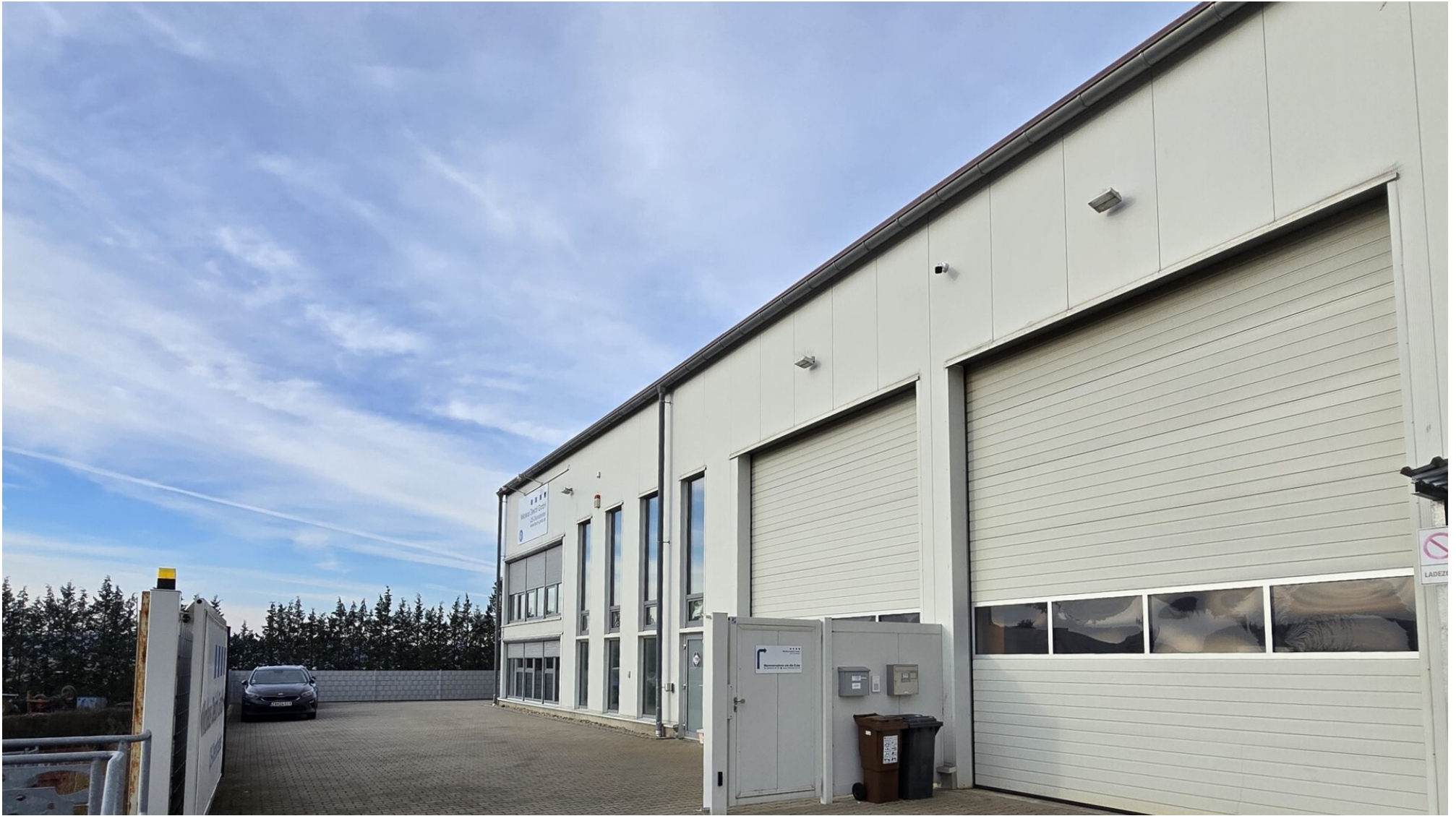
BI-25-02_SW 10 Halle Ost-West
